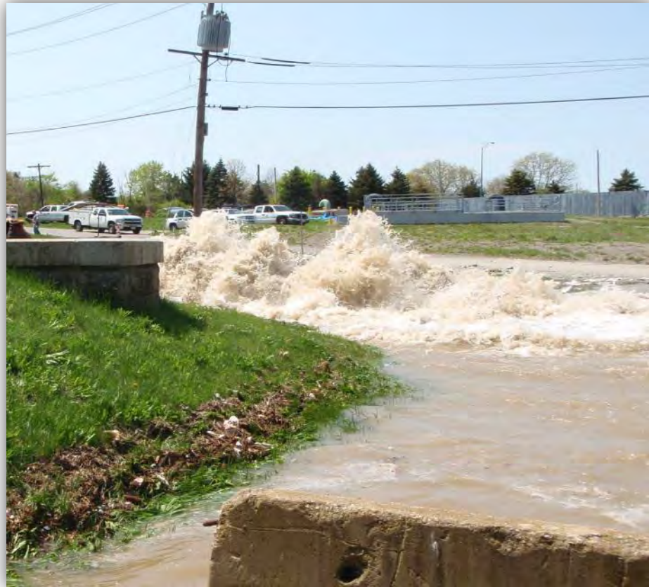
250 MGD flow at Shaft 5 break....
