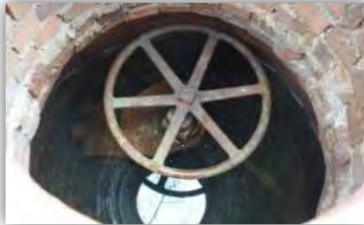
Shaft 7C connection to Section 58
